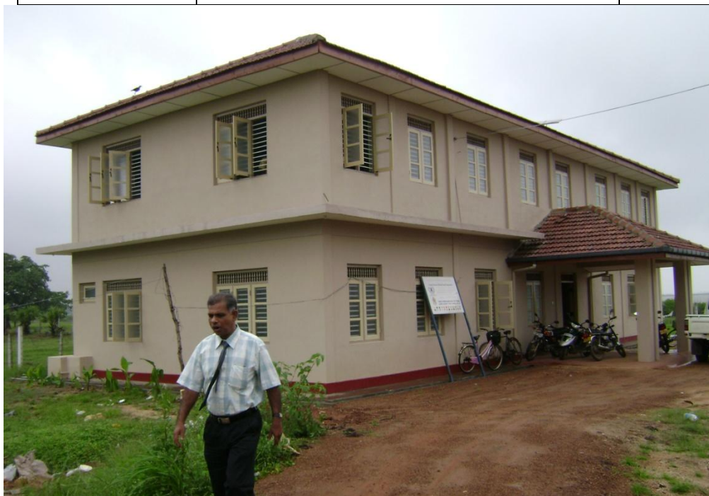
Newly constructed of MOH Office at Vavunathivu in Batticaloa - under WB/HSDP
